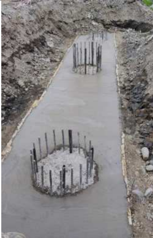
Bridge construction works above the amelioration canal
