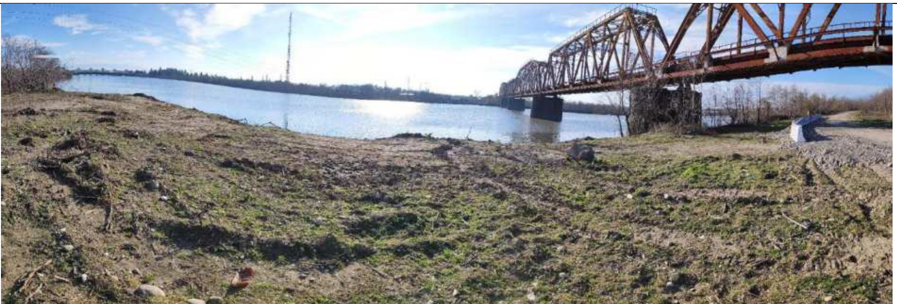
Panoramic view of the bridge pier location near the Rioni river (looking southeast)
