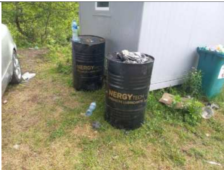
Improperly stored hazardous material containers
