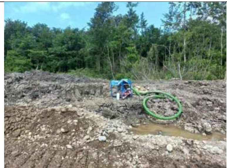
Water pumping from the small ponds in the eastern part of the project
