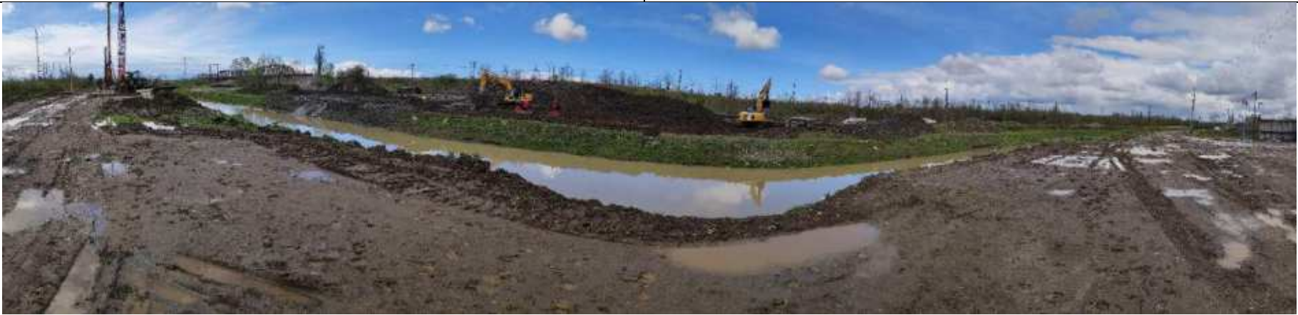
Panoramic view from the gas relocation works and amelioration canal
