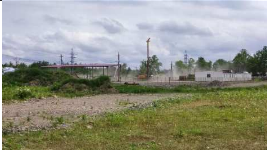
Dust generated during heavy construction machinery movement
